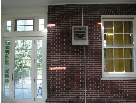
Sun Porch, North Wall
