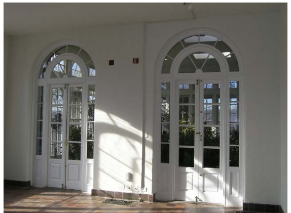
Sunroom, West Wall, with doors to Sun Porch
