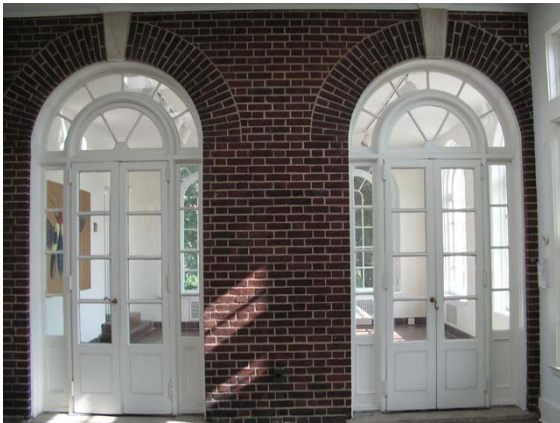
Sun Porch, East Wall, with doors to Sunroom
